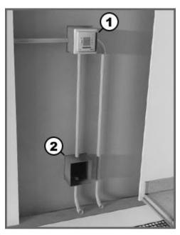
**6.** Measure the insulation values with a Megger (Insulation Resistance Meter) tester and record the value (see page 17). Make sure there is no insulation problem.
